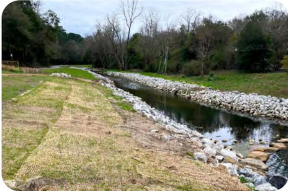
**Streambank stabilization in Langan Lake Park reduces the erosion that has historically impacted the lake.** Credit: RESTORE Council
